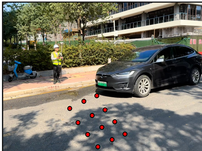
Hazardous location- Road Site
