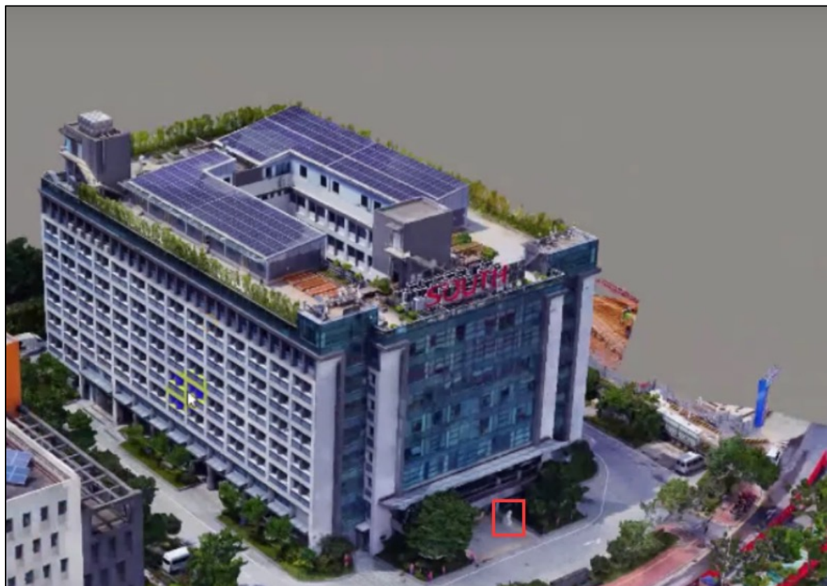
UAV Survey for SOUTH building, Lion statue detail lost
